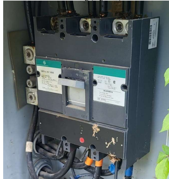
Figure 2 - Utility power enters the building at 101 through this breaker box.
