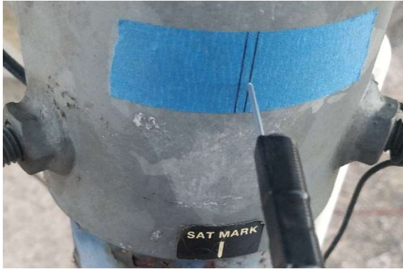
My reference marks and pointer for rotating the antenna to the new azimuth.
