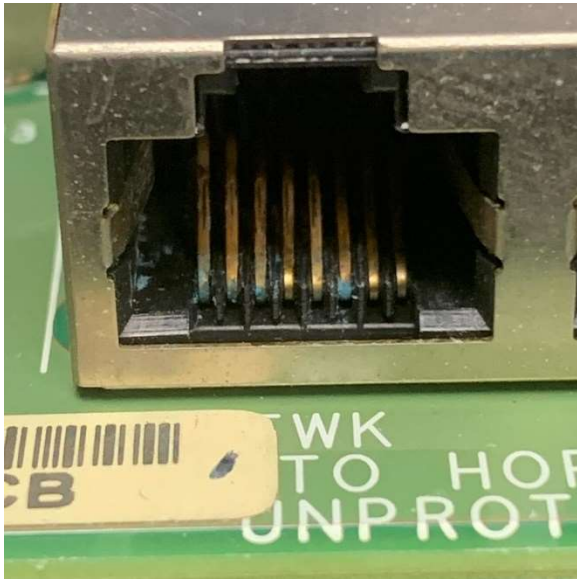
Figure 3 - Hidden corrosion was causing an intermittent link.
