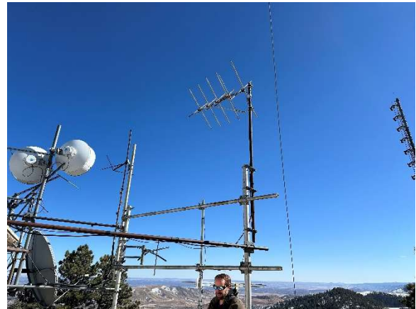
The finished product... the Kathrein-Scala CA5-FM/CP/RM looks out over Denver metro from 7,383 feet AMSL (2,100 feet above the city).
