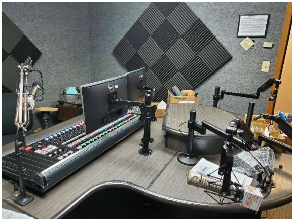
LXE/Wheatnet installation in progress in one of the control rooms.
