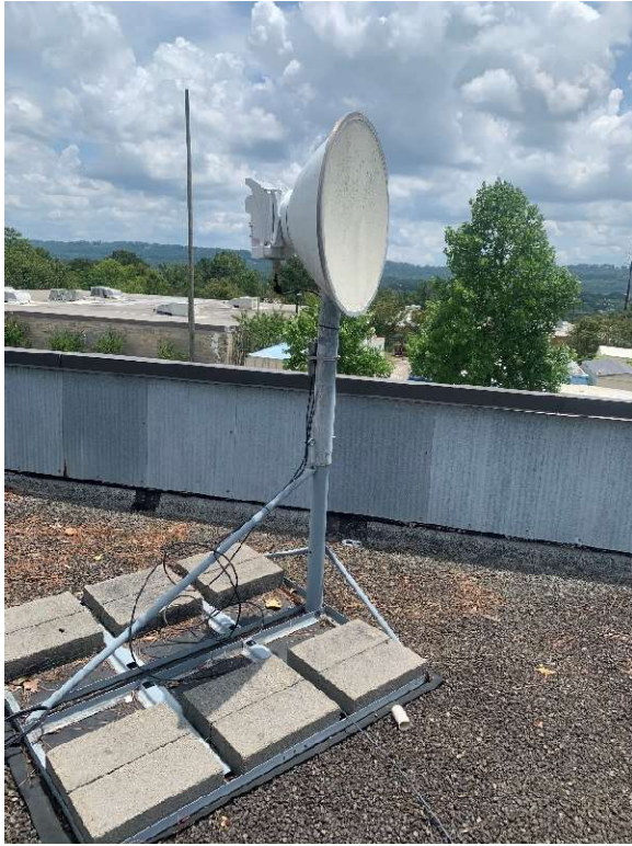
The 18 GHz antenna on the studio roof is now on a much more secure mount.
