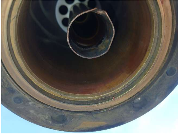
The interbay just above the power divider tee in the Shively aux. Somebody split a bullet when the antenna was installed.
