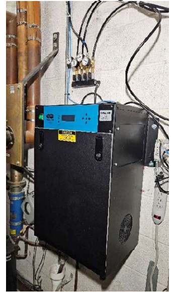
Our Altec Air pressurization system.
