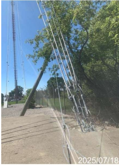
The broken pole that was supporting part of the WRDT night ground cables.
