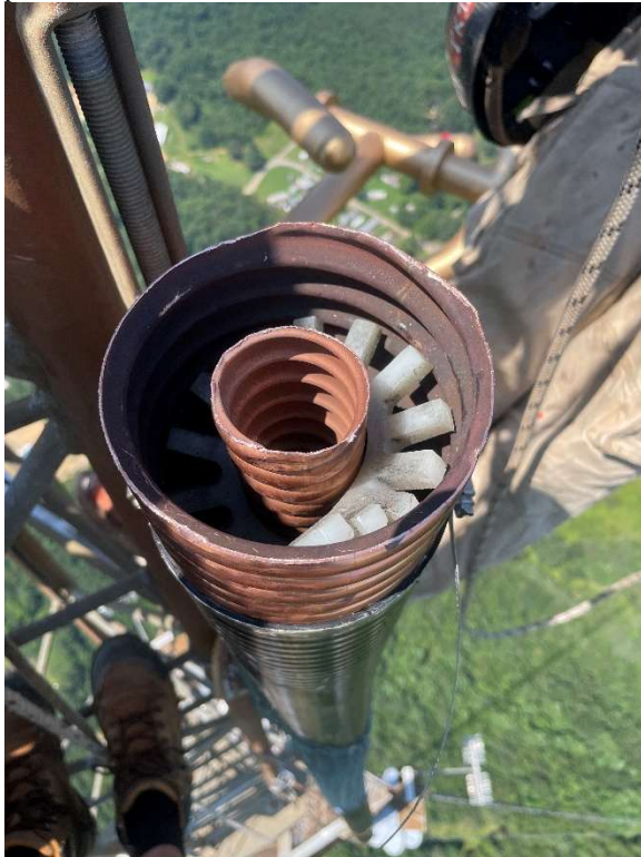
The end of the line before the new connector was installed. Not too bad but not pristine.
