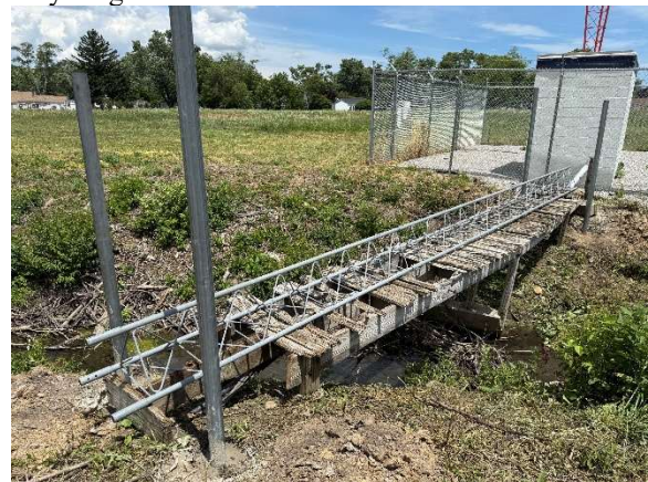
Figure 2 - The new bridge under construction.
