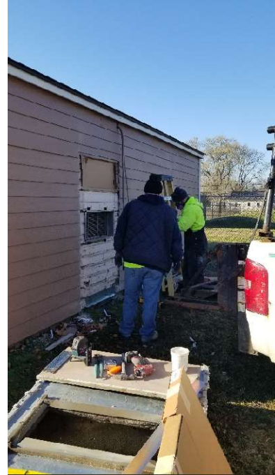
Installing the new HVAC unit at the WCHB site.
