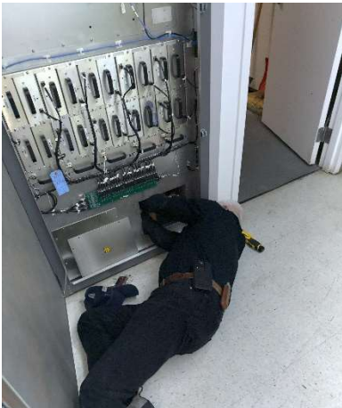
The old man helping me out with re-tapping the NX50 transformer. I couldn't reach the back (front, really) taps from the rear.
