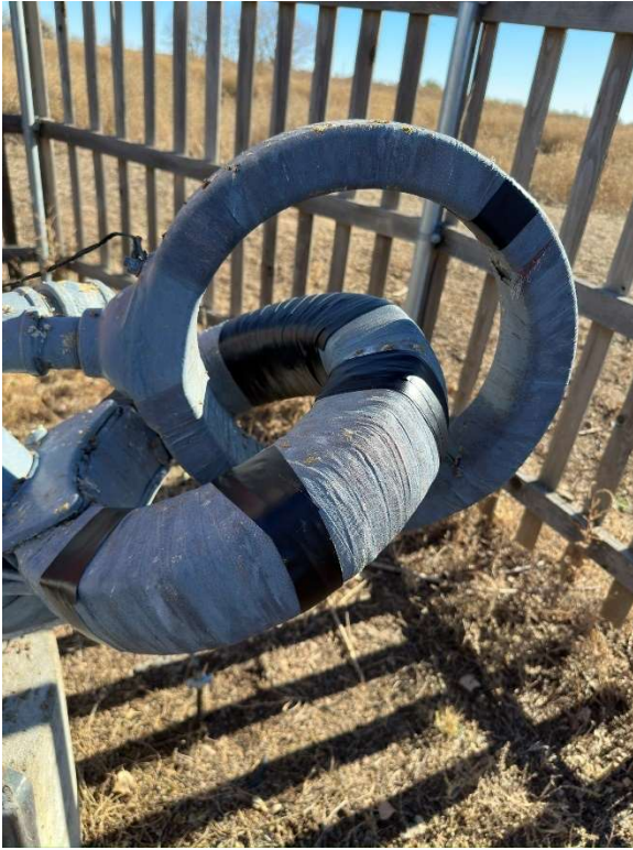
The Austin Ring primary was taped up to keep water out of the windings until we can completely rewrap and epoxy paint the whole thing in the spring. We've got several of these to do.
