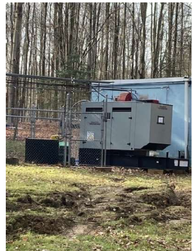
All dressed up with no place to go, the new generator is sitting pretty sans transfer switch at the WDCX-FM site.
