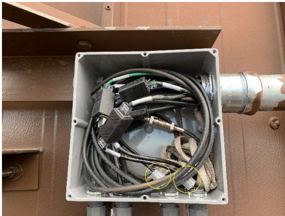
Figure 1 -- A couple of clamp-on ferrite cores are visible in this rooftop junction box. The others are hidden behind wiring and pull-tape in the box, but every cable in the box has a ferrite installed. Here we employ belt and suspenders -- the CAT5 is also shielded and in conduit! Why take a chance?
