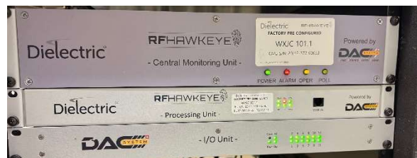
Figure 2 – Along with the line section, this hardware continuously monitors the transmission system from the transmitter building to the top of the antenna.
