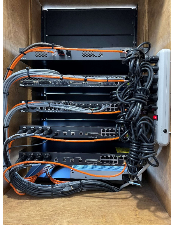
The KLZ blade stack from the rear. By the time you read this, the bundled power cables will have been replaced with 1-foot EIA cables.
