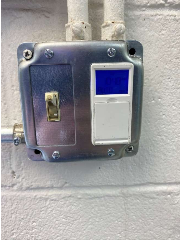
The new timer switch at the KLTT transmitter site. Yes, the interior light switch is THAT dirty!
