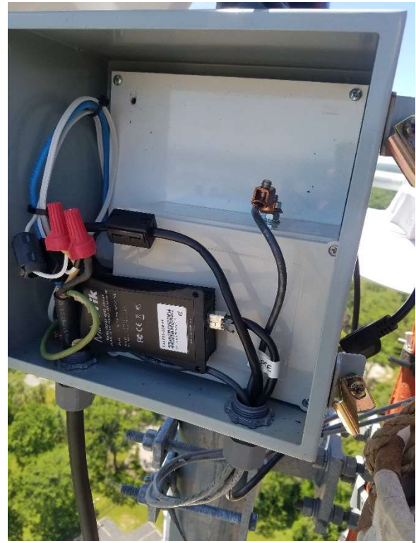
A much neater installation on the WMUZ tower: The gray box is the POE/suppressor for the Trango Apex Lynx microwave radio on the tower at the WMUZ studio. The black device is a 48-to-24 volt converter for the Ubiquiti Powerbeam radio.
