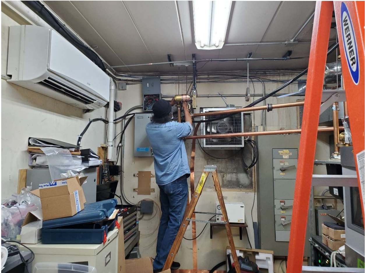
James fits a 3-1/8" elbow for the WPWX offsite auxiliary at the Lansing site.
