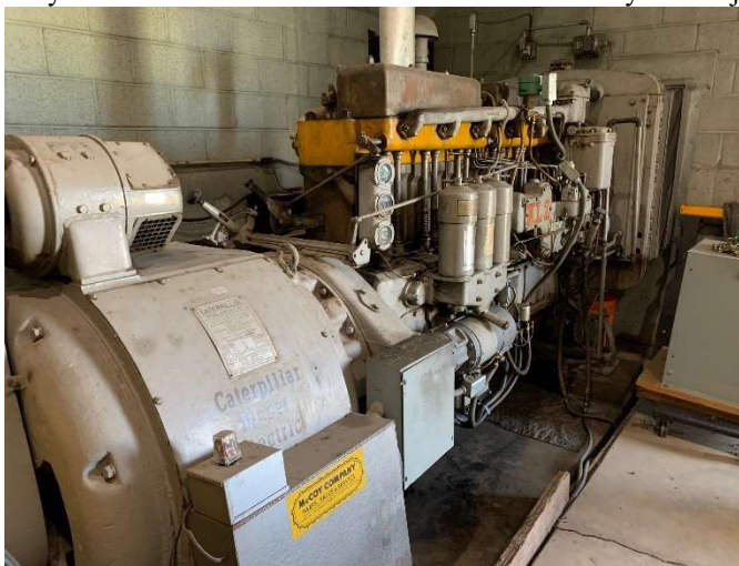
The 1946-vintage Caterpillar generator at the KLZ transmitter site.
