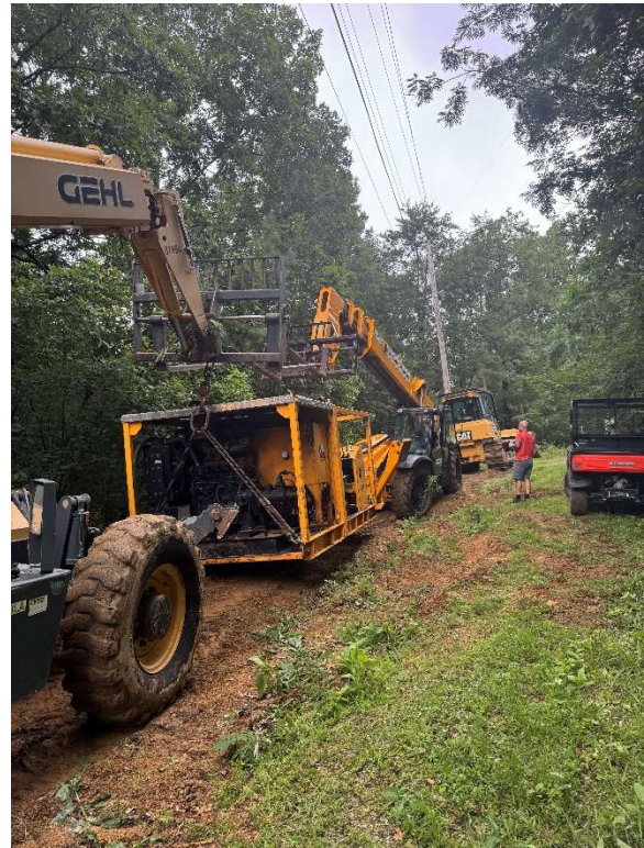
It took a dozer pulling a lift with another lift behind to get the mammoth winch up the hill to the WXJC-FM tower site. The ground was so wet the lifts could not move the winch by themselves.
