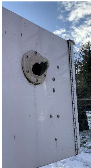
Figure 1 - Broken bowl insulator on the 1640 ATU/filter cabinet.
