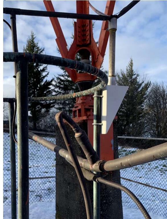
Figure 2 - Mangled feed tubing at one of the towers.
