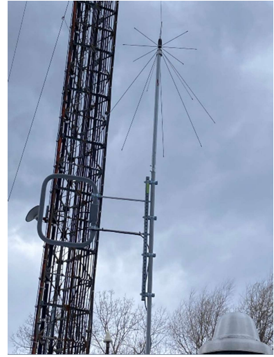
AM loop and "Disk-cone" FM receive antenna at the WLGZ-FM site.
