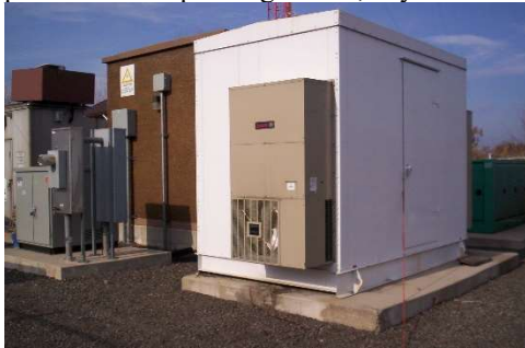
The 150 kVA 480 VAC flywheel UPS at Crawford's WPWX site in Burnham, Illinois is housed in this standalone, self-contained shelter. It features dual HVAC units and bypass switching.
