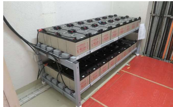
A UPS battery bank at an American Towers site.
