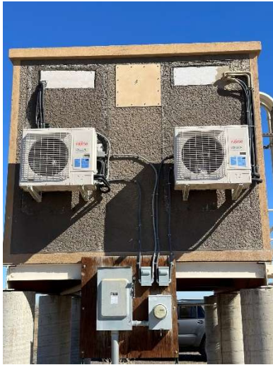
The two new Fujitsu 3-ton A/C units on the KLVZ transmitter building.
