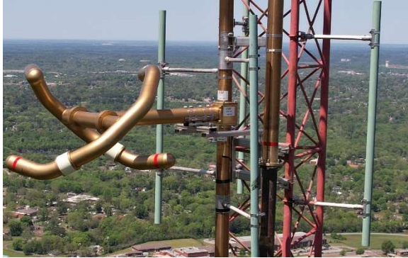
Figure 1 – Look closely at the lower saddle clamps holding the directors to the interbay line. Not just no...
