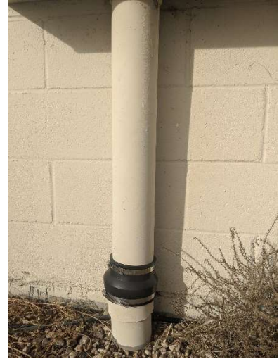
The fix is in on the 5-inch conduit at KLTT.
