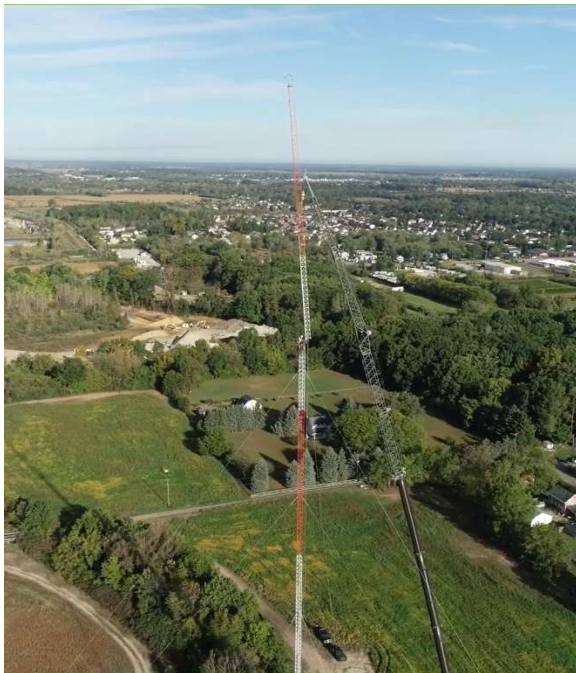
The 393-foot reach crane had just enough to set the top sections in place.
