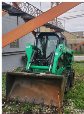
Larry used this Bobcat to remove the rock and dig the hole.
