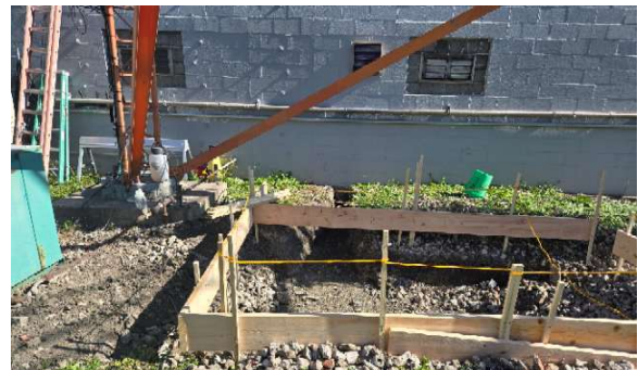
Almost ready for concrete. We still need to run the conduit.
