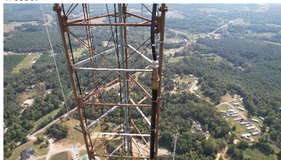
The point 200 feet below the antenna input where the new 3-inch line section is connected.
