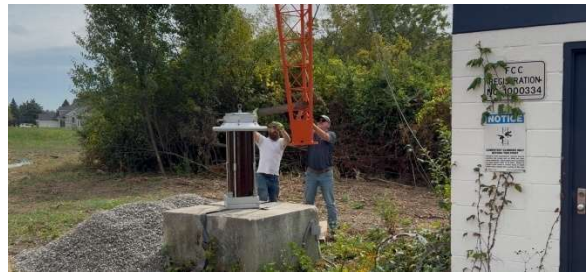
Figure 2 - That is one big base insulator!
