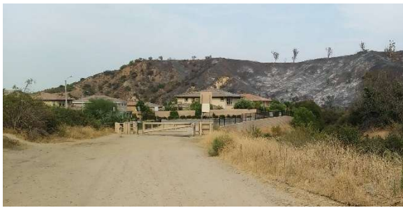
The area around the Skyline Drive entry gate below the KBRT transmitter site. Note the burn scar behind the houses.
