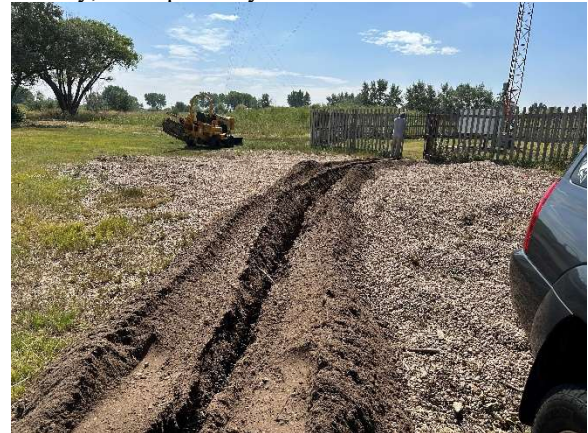
The trench to KLTT tower #1 for the new control and power cables.
