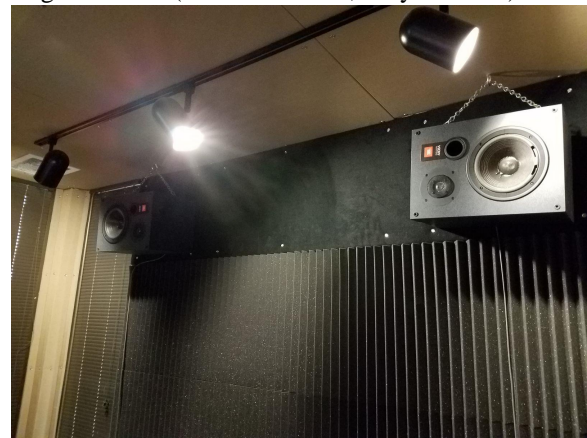
Figure 4 - WDJC's control room. Still a work in progress, but it sounds (and looks!) much better!
