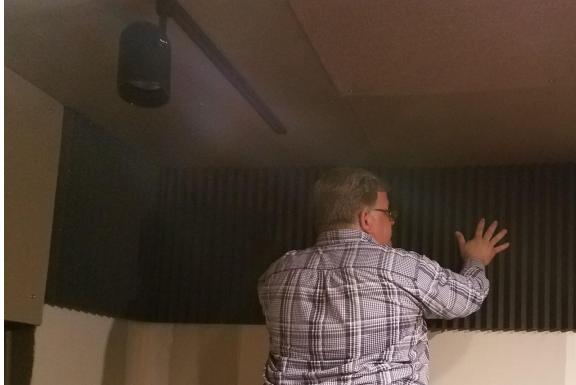
Figure 3 - Todd installing some of the Auralex Studiofoam in one of our production rooms.
