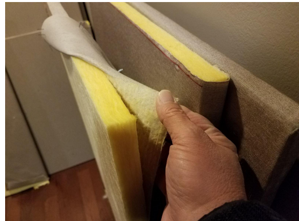
Figure 2 - The (not very absorbent) cloth was glued onto the foil side. Totally ineffective.
