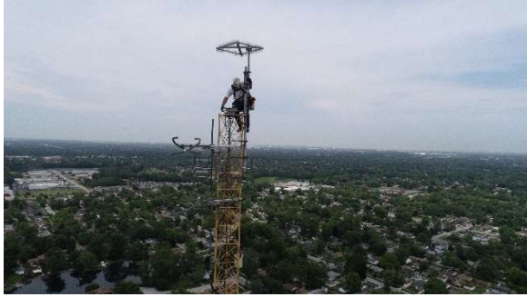
A tower worker installs a new flash head on top of the Lansing tower.
