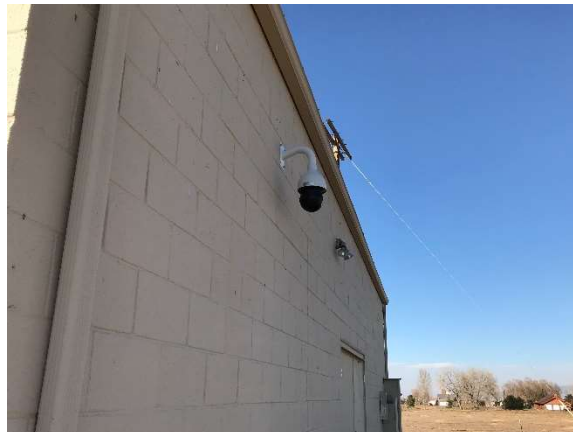
This 1080 PTZ camera gives a complete view of the KLTT antenna field, providing close-ups of all the tower base areas. Amanda can even use it to observe the tower lights operating.
