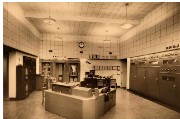
The pre-fire KPOJ transmitter facility at Mt. Scott.
