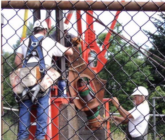
The P&R crew hoists the replacement insulator into place at KKPZ.
