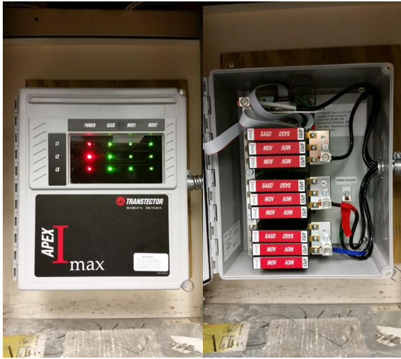
Front and inside view of the Transtector Apex I Max
