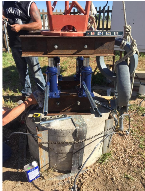
KLTT Tower #2 up on four bottle jacks during base insulator replacement.
