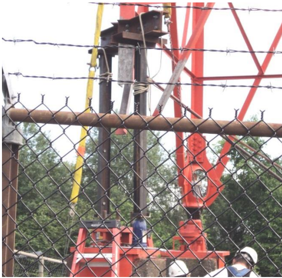
KKPZ tower with one of the insulators removed and jacks supporting the leg.
