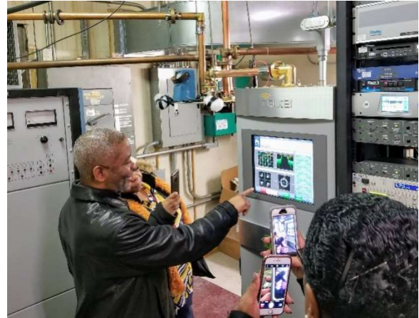
WSRB PD Jay Alan turning the new transmitter on.
