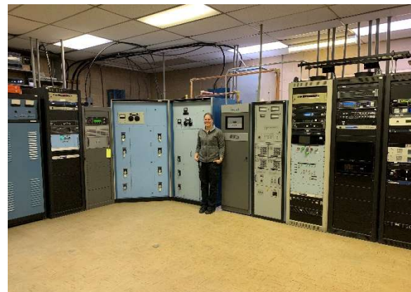
A panorama of the completed KLZ transmitter room. Left to right, the AMPFET 10 (not connected), the KLDC night rack, the KLDC night J1000, the KLDC night four-tower phasor, the KLZ phasor, Amanda, the new KLZ NX5 main, the ND5 aux and the three KLZ equipment racks.
