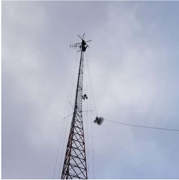
Figure 1 - 1260's new Cambium headed up, the old Trango coming down.
