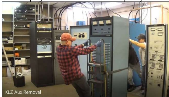
The old man helps Amanda and Keith horse the old AMPFET 10 out of its slot and across the room, making room for the new NX5 at KLZ.
