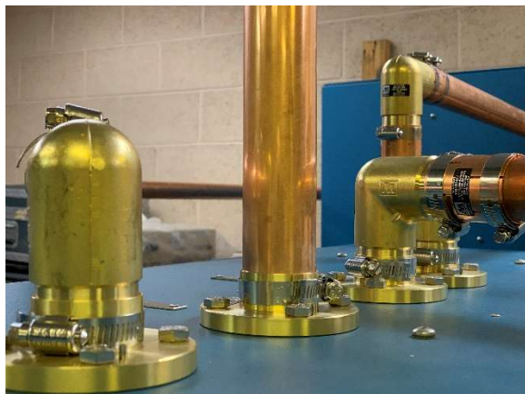
1-5/8" EIA RF plumbing on the top of the KLZ phasor. The dummy load is visible on the wall behind the phasor.
