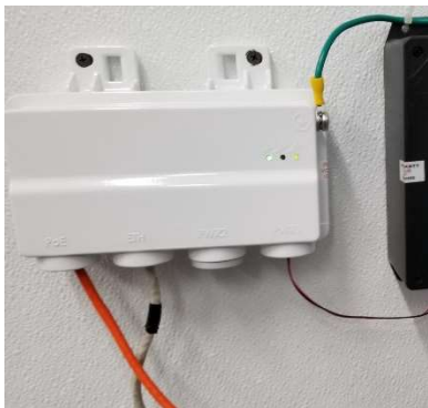
Figure 2 -- Cris ordered this shielded, grounded power injector for 1260.
