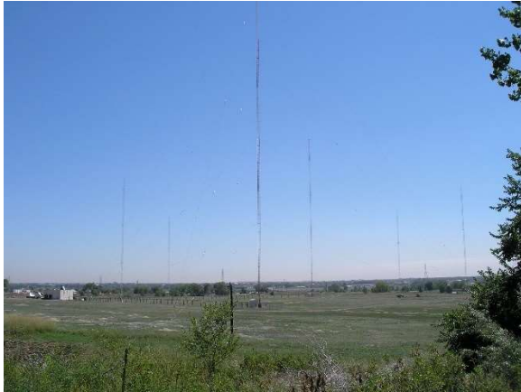
The KLZ transmitter site. Note the two tall (450-ft.) towers, four short (200-ft.) towers, and the above-ground line supports to the two tall towers.
