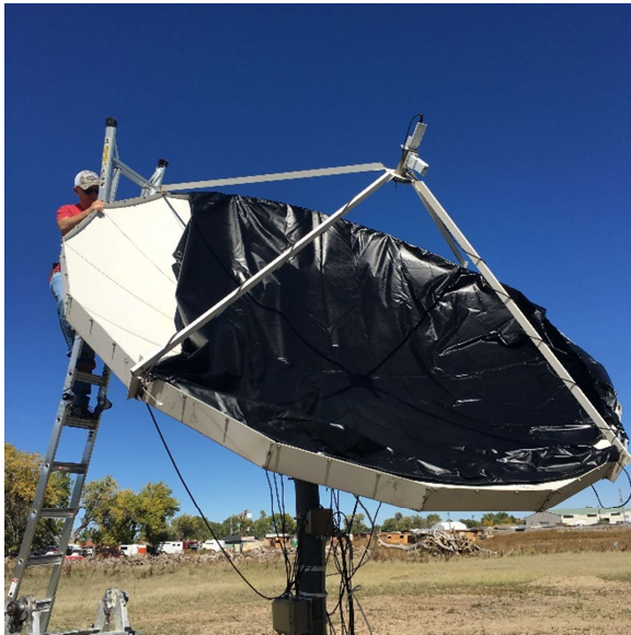
My husband, Jordon, helps install the snow cover on the KLZ C-band antenna.
