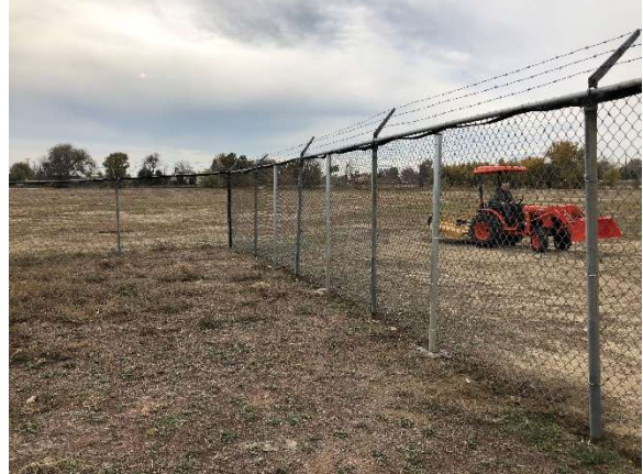
The repaired fence with shiny new posts.
