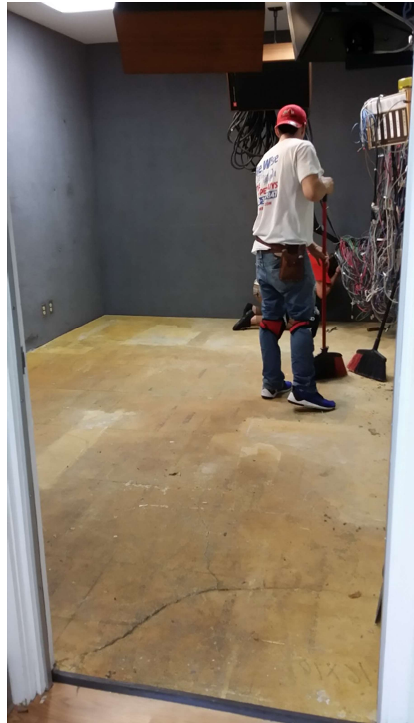
The WMUZ-FM control room cleaned and ready for new carpet
