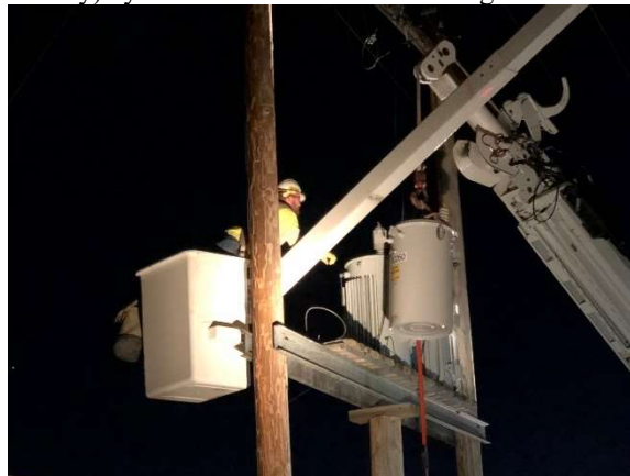
United Power replaces a 100 kVA transformer at the KLTT site.
