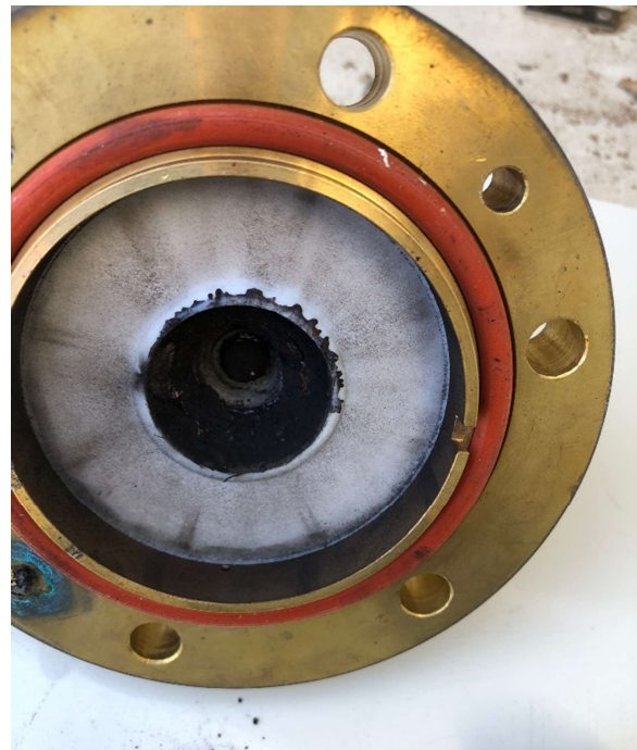
Burned out end terminal adaptor from KLTT tower #1. Note that the Teflon does not show signs of arc-over.
