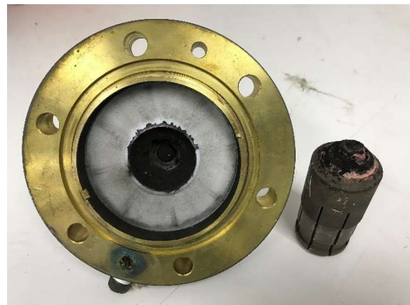
The damaged end terminal adaptor -- note that the stud on the back of the bullet has been vaporized.
