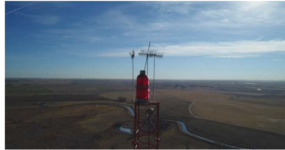
Figure 1 - KLTT tower 2 -- the lightning rod is loose.
