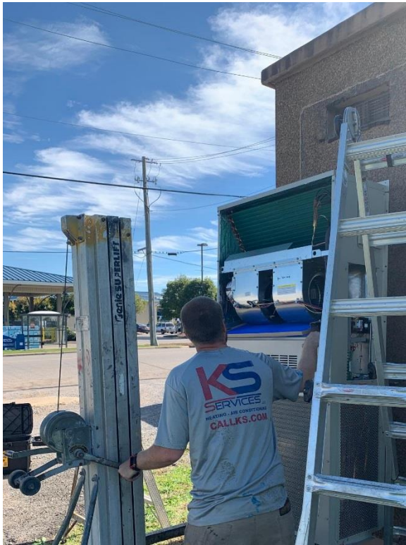
Figure 1 - Lifting the 3 ton unit into place at 1260.
