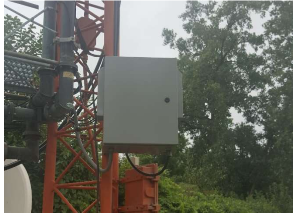
48-VDC UPS mounted on a tower leg at WMUZ.
