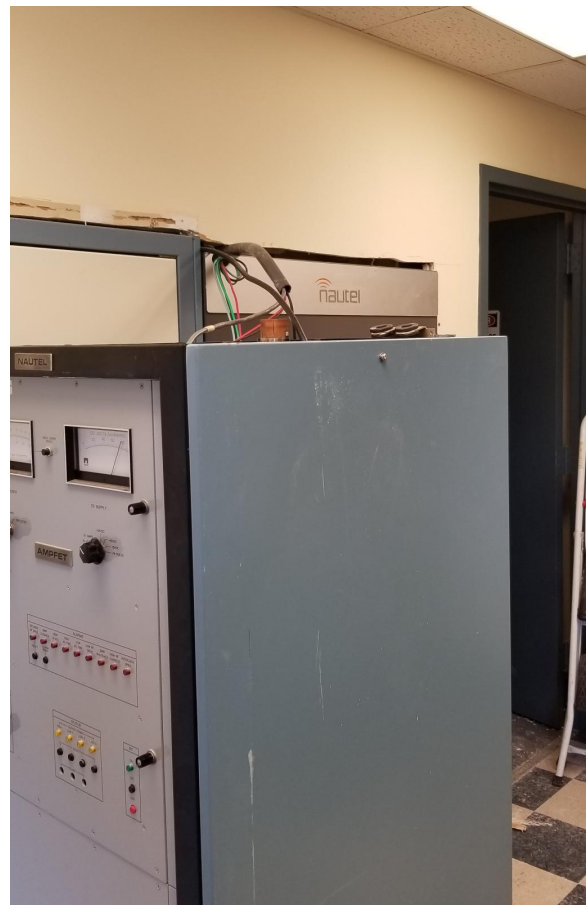
Figure 9 - Temporary rigging of the old night transmitter.
